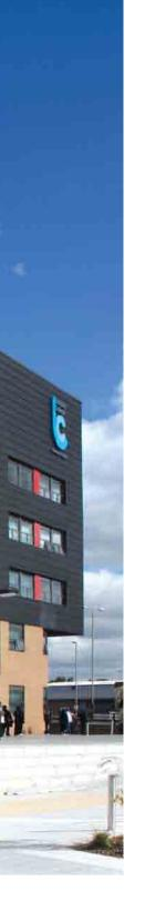
SCW curtain wall has been designed to meet current building regulations. It is a semi-unitised, zone drained and pressure equalized system and offers a slim 50mm sightline, with a choice of three mullion and four transom depths.
